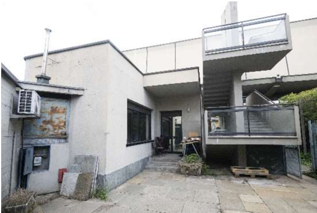
Figure 4-14 Exterior of the former Caretaker's House
