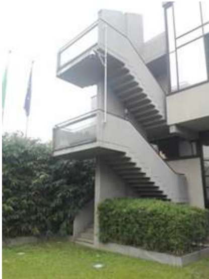
Figure 5-7 Staircase 1, serving the Library and Photographic Archives
