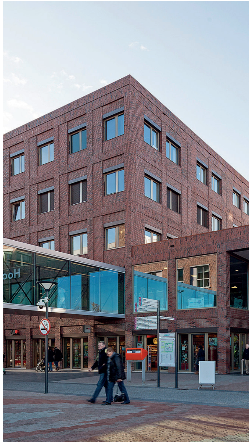
Maasstad Hospital, Rotterdam, The Netherlands (2011)
