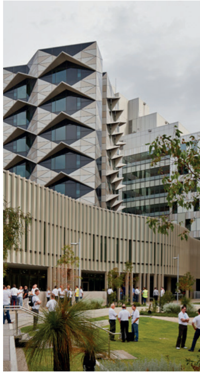
Fiona Stanley Hospital, Perth, Australia (2014)
